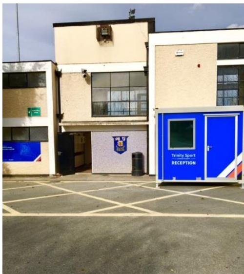
Office at Santry Sports Grounds
