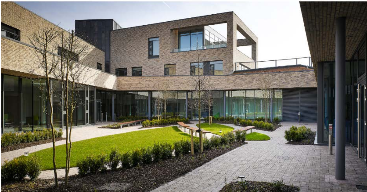
07: Phoenix Care Centre, Grangegorman, Dublin 7, Dublin.
