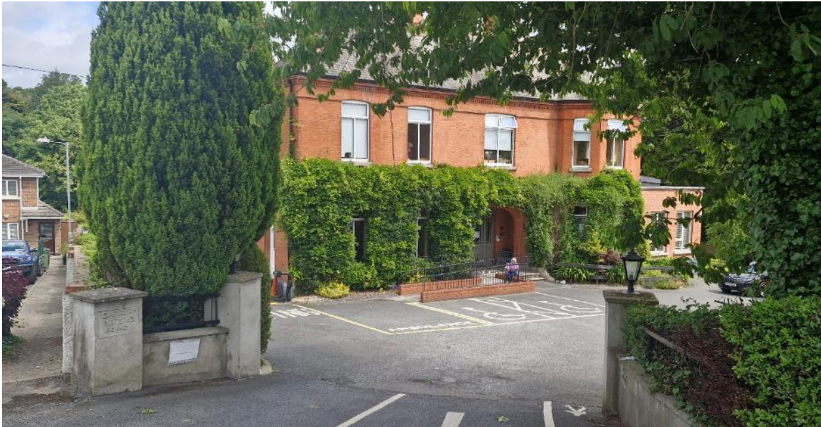
06: Glenaulin Nursing Home, Chapelizod, Dublin 20, Dublin.
