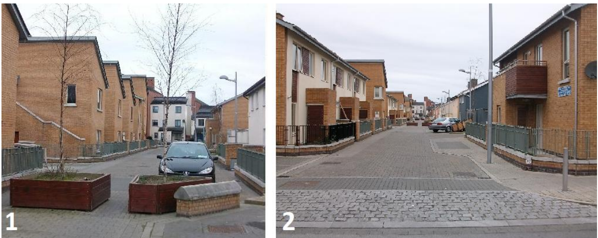
Figure 9.12.B – Design features of Dolmen Lane Home Zone.– 1 – planting. Image 2 – Horizontal deflection
