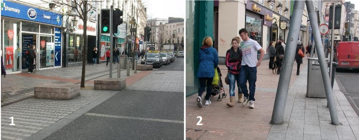
Figure 9.6. B - Patrick Street in Cork. Image 1 – Kerbless edge / level surface . Image 2 – lighting stands
