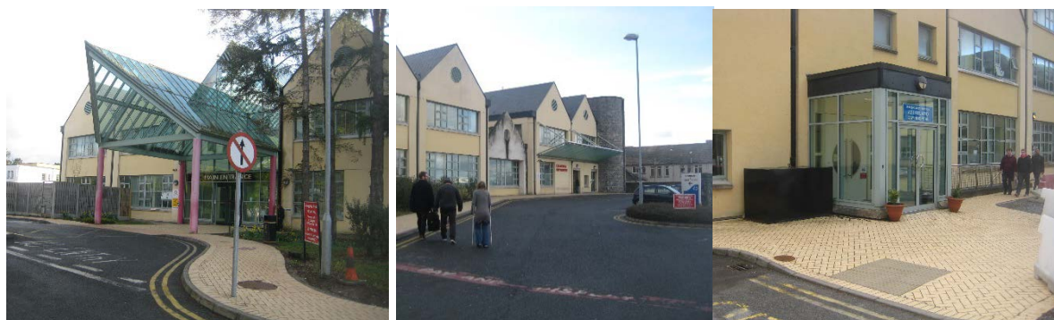
Figure 7.21: Main entrance (left), ED entrance (middle), Day Hospital (right).
