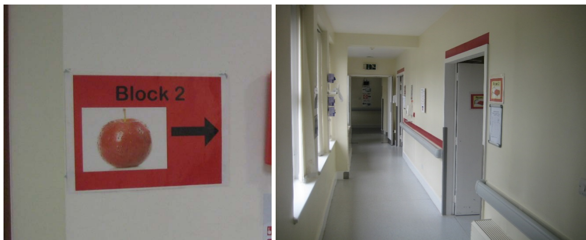
Figure 7.42: Wayfinding signage with colour and symbol (left) colour-coding on doorway into ward (right).
