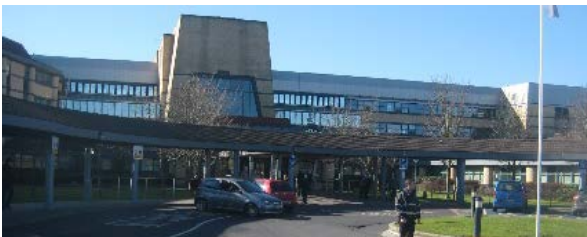
Figure 7.4: Main Hospital Entrance.
