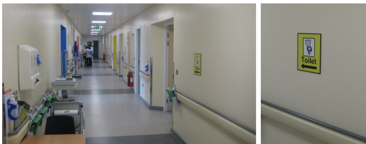
Figure 4.24 – Corridor in Rowan ward showing yellow toilet signage and yellow reveal to toilet door (left) and close up of toilet signage (right)
