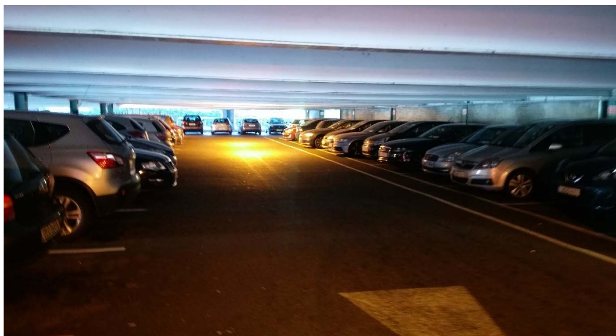
Figure 7.43: Multi-storey carpark in Tallaght.
