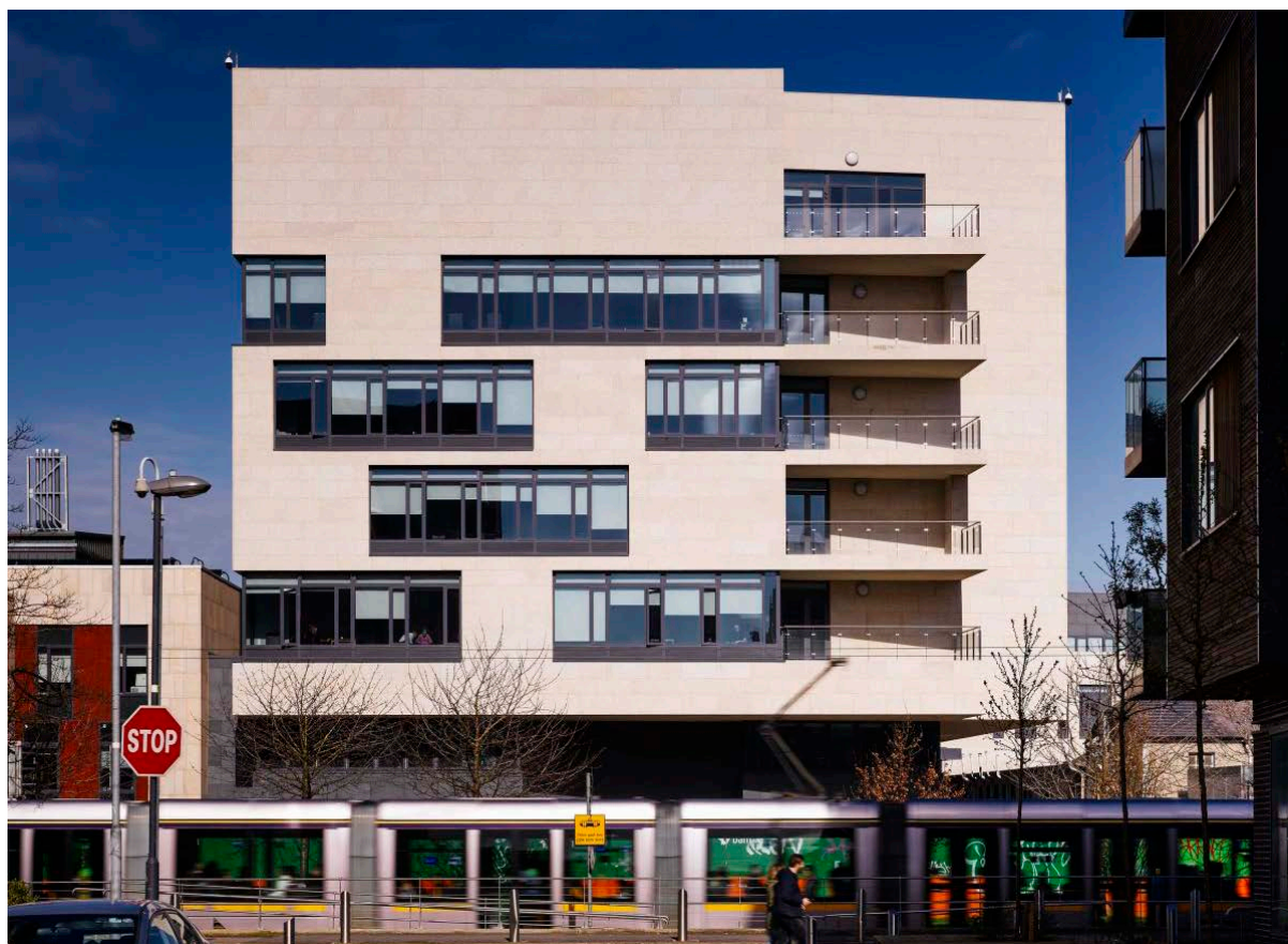
Figure 4.3 – View to front of the MISA building showing the adjacent Luas line
