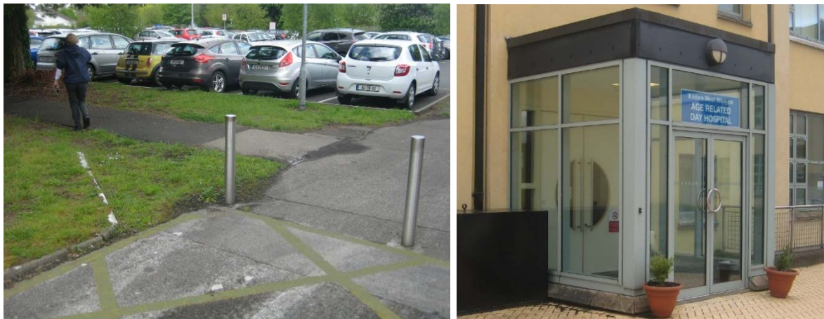
Figure 7.29: Onsite footpaths (left) entrance door to the Age-related Day Hospital (right).
