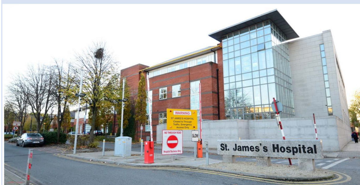
Figure 4.2 – View to front of hospital
