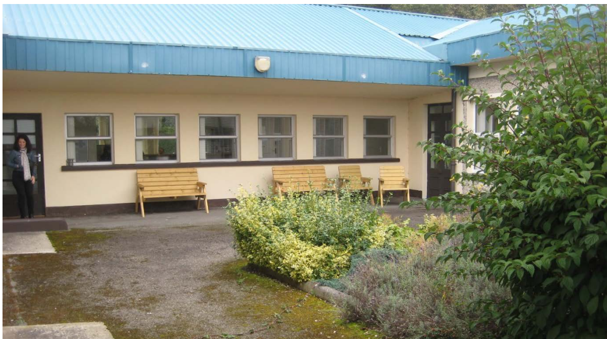
Figure 7.39: Internal courtyard with eating and planted areas
