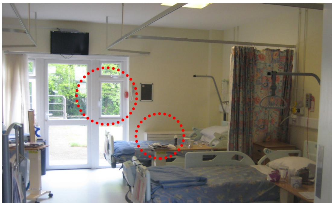
Figure 7.44: Opening windows and flat panel radiators in-patient wards.
