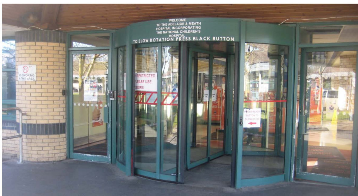
Figure 7.14: Main entrance door- Central revolving door with swinging doors either side.
