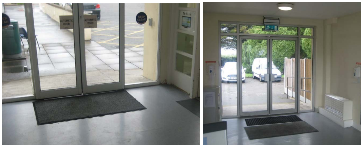
Figure 7.40: Electric doors, main entrance (left) rear doors (standard hinge) (right).
