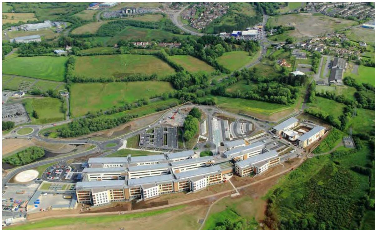
Figure 6.2: Aerial view of South West Acute Hospital in Enniskillen
