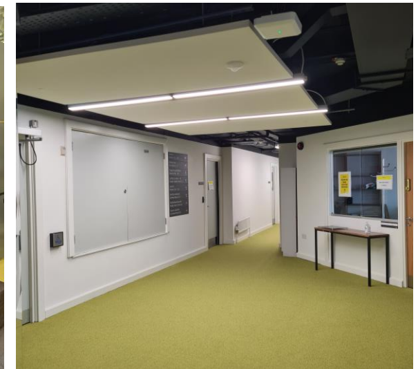
Aras an Phiarsaigh: LED lighting with occupancy controls (photo: Kieron McGovern)
