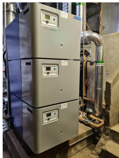
Chemistry & Anatomy Buildings: Boiler upgrade front (left) and back (right) (photo: Kieron McGovern)
