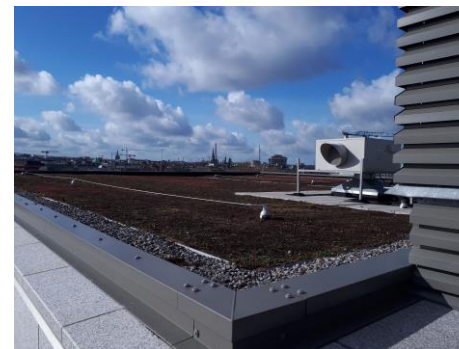
Sedum green roof to attenuate surface runoff
