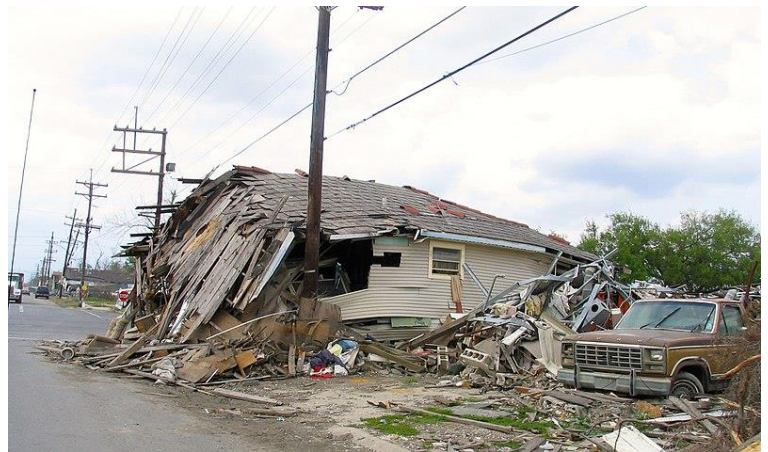
Damage from Hurricane Katrina to New Orleans - taken seven months after the hurricane (image by: Gregory Varnum) (Licence: https://creativecommons.org/licenses/by-sa/3.0/deed.en )
