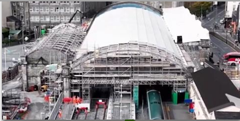
Galway station is being redeveloped
