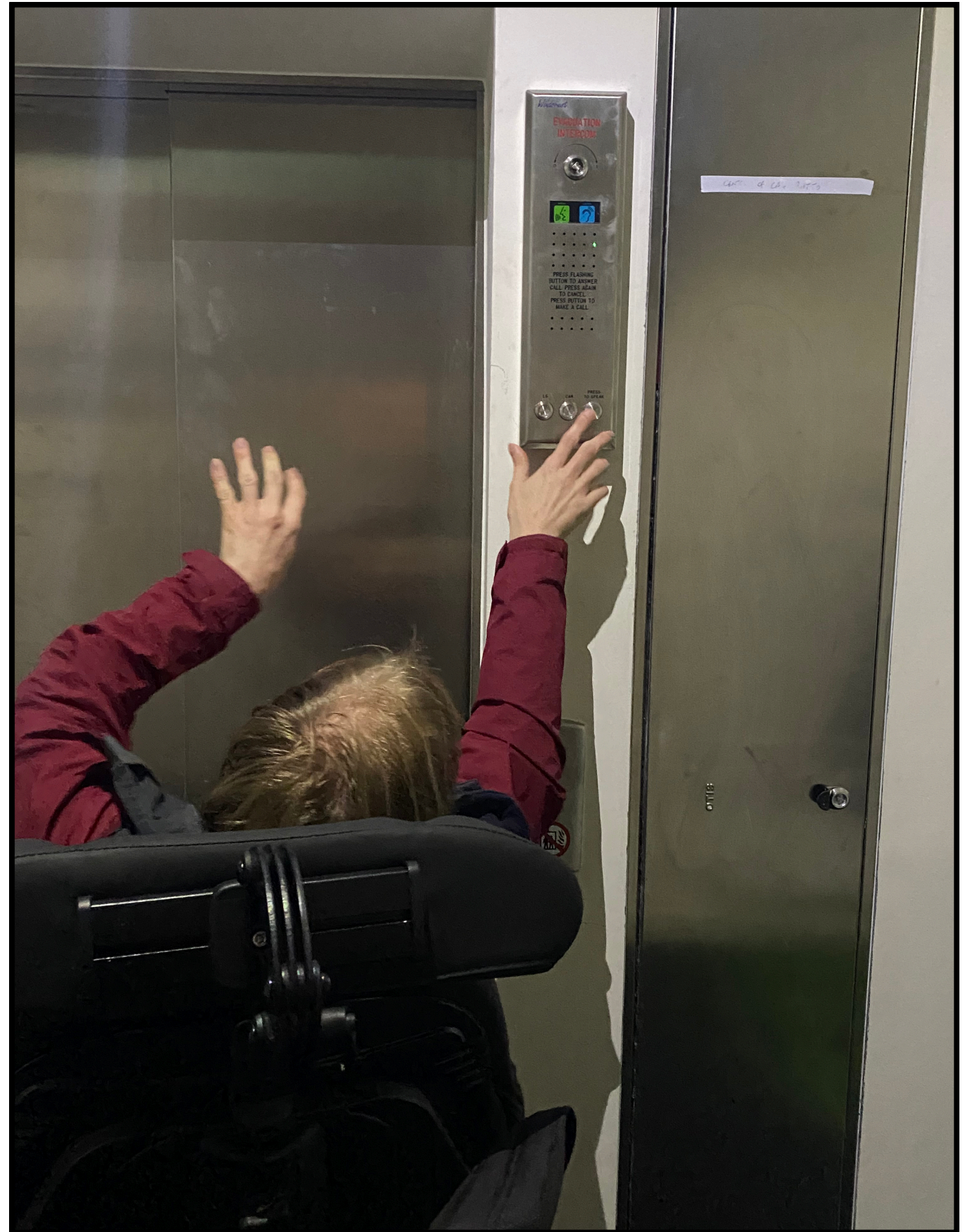
Figure 22 - Printing House Square. Lift controls and emergency intercom positioned too high, making them difficult to reach for wheelchair users.
