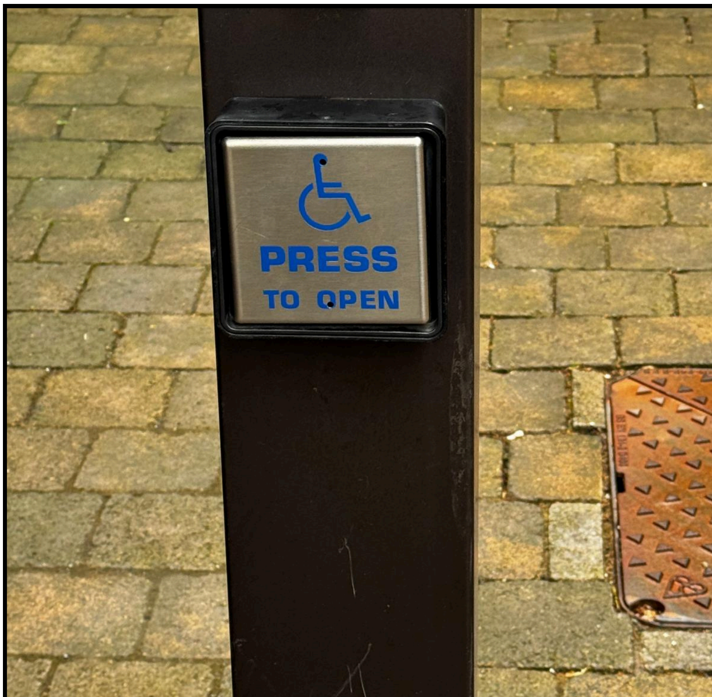
Figure 11 - Clearly visible and accessible push-button control supporting independent entry.
