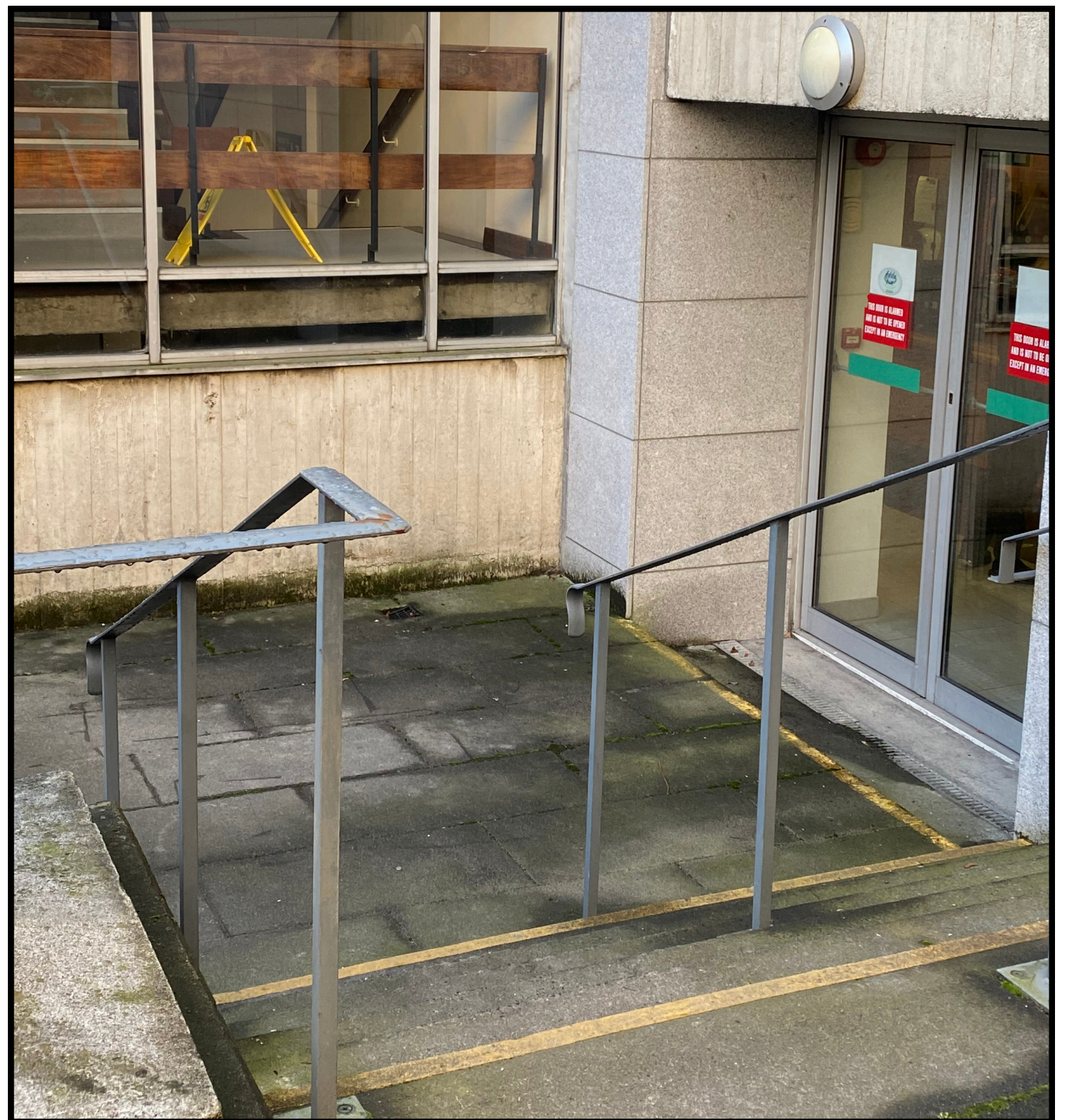
Figure 16 - Entrance to Seomra na Gaeilge with step-only access and no step-free alternative, creating an exclusionary design.
