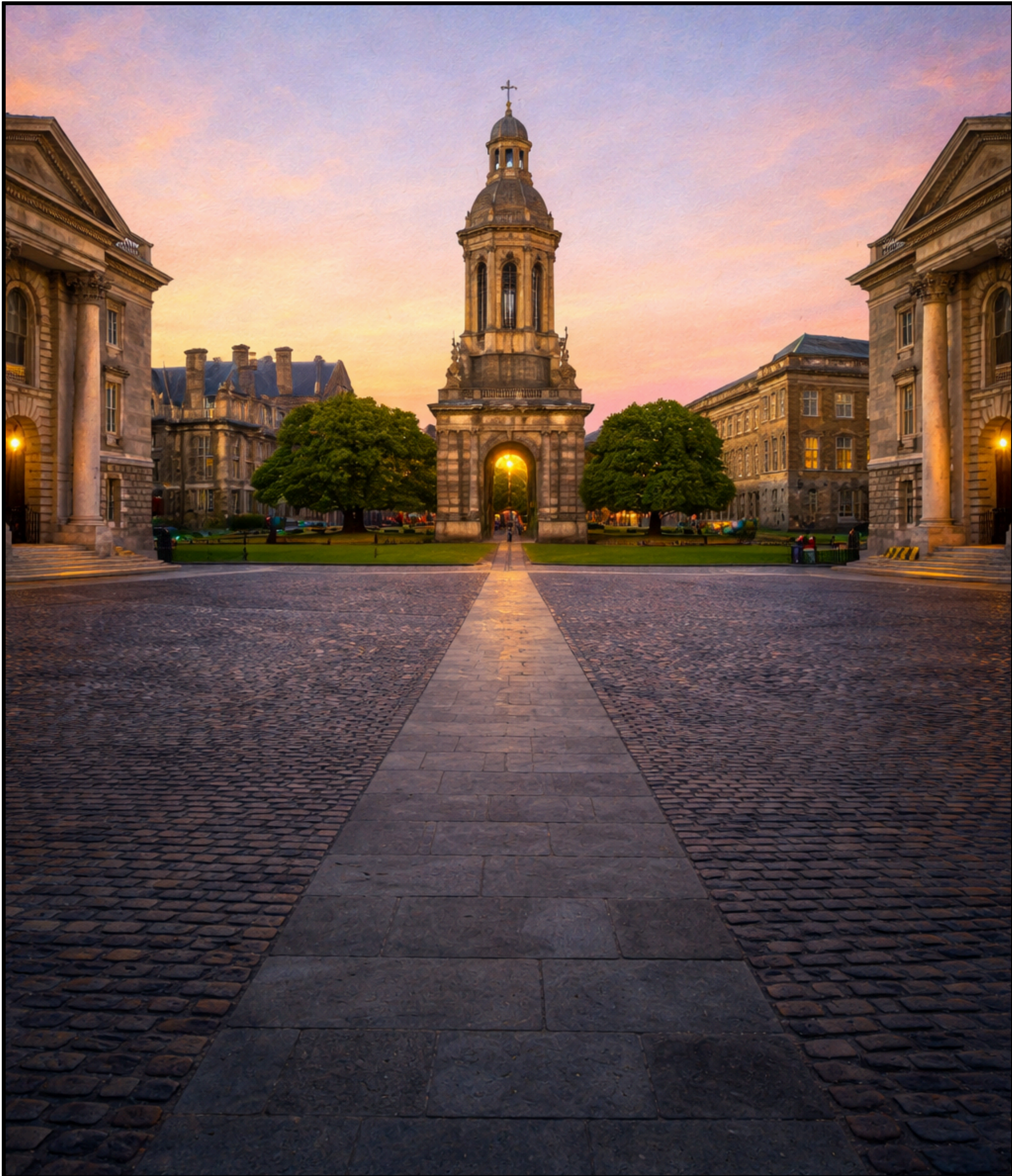
Front Square and the Campanile, with the accessible pathway that supports legibility, orientation, and independent access.
