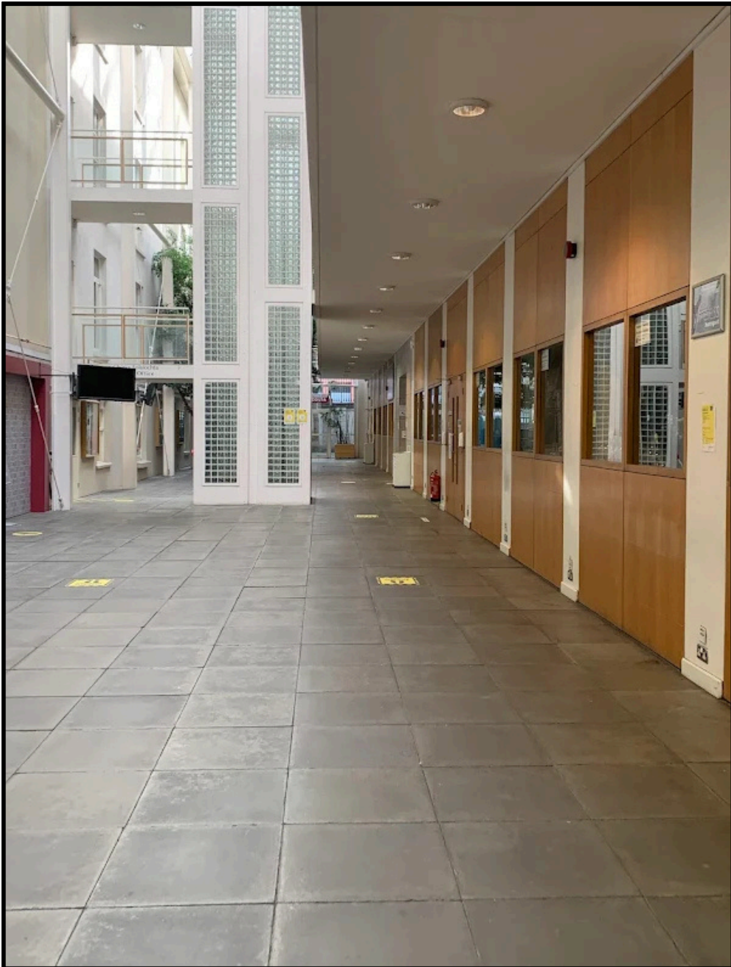
Figure 19 - Hamilton Building. Wide, unobstructed internal circulation route supporting clear and independent movement throughout the building.
