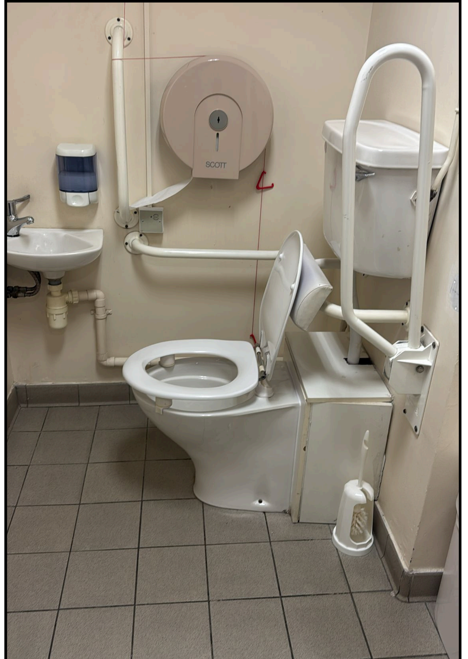
Figure 30 - Emergency assistance cord tied above floor level, preventing safe use in an emergency.
