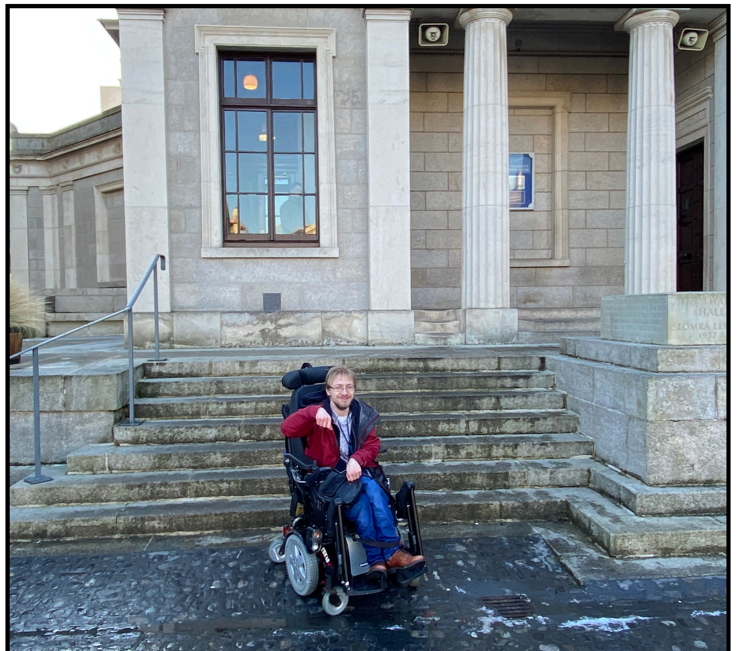
Figure 7 - Step-only entrance to the 1937 Reading Room, preventing access for wheelchair users.
