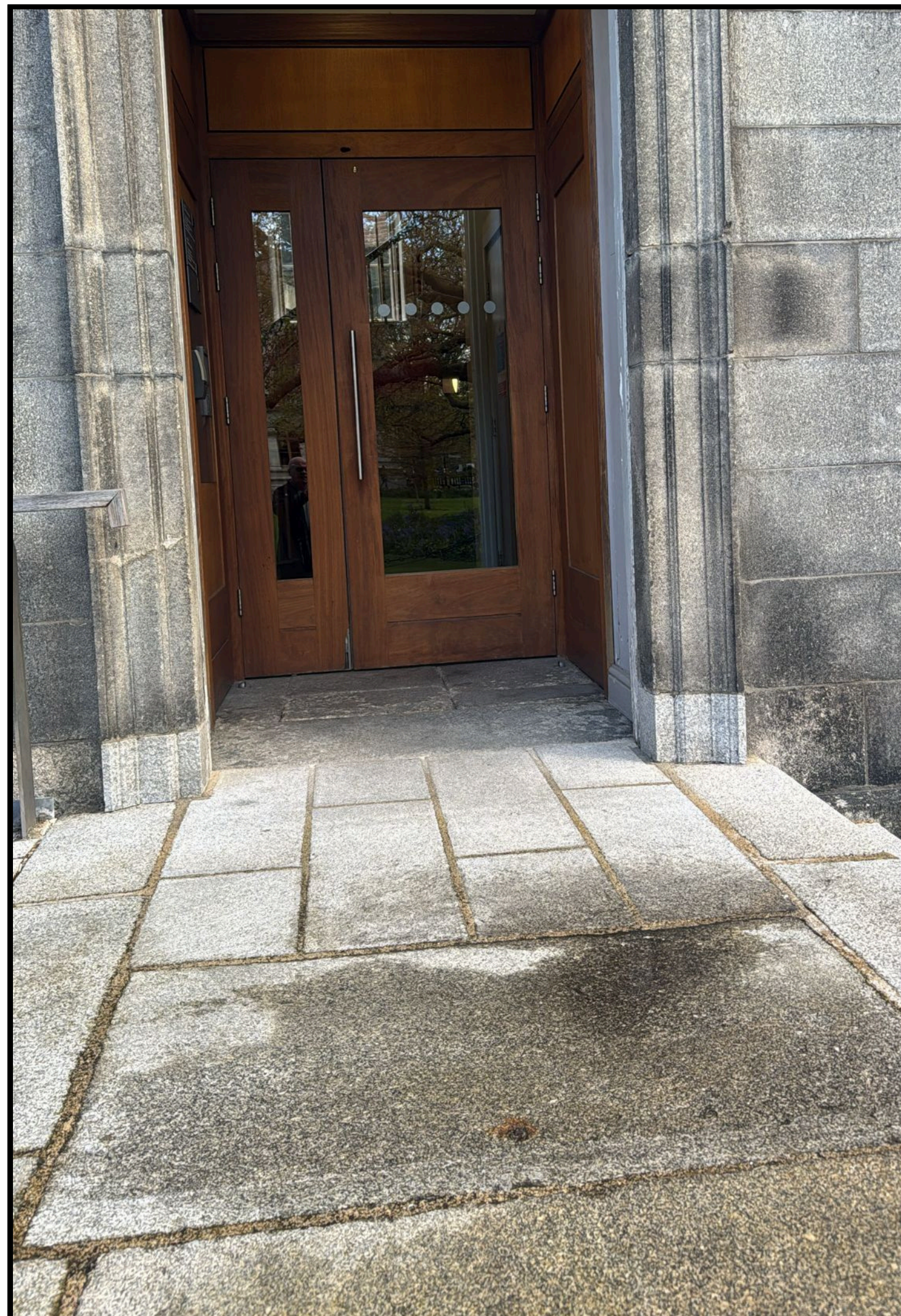
Figure 14 - Entrance without automatic door, limiting independent access for some users.
