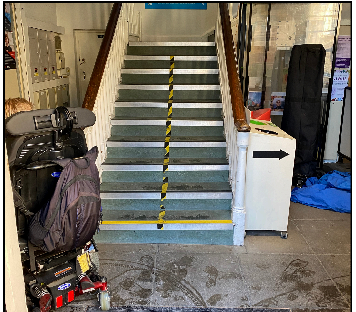
Figure 9 - Step-only entrance at House 6 with no step-free access, creating a barrier for wheelchair users.
