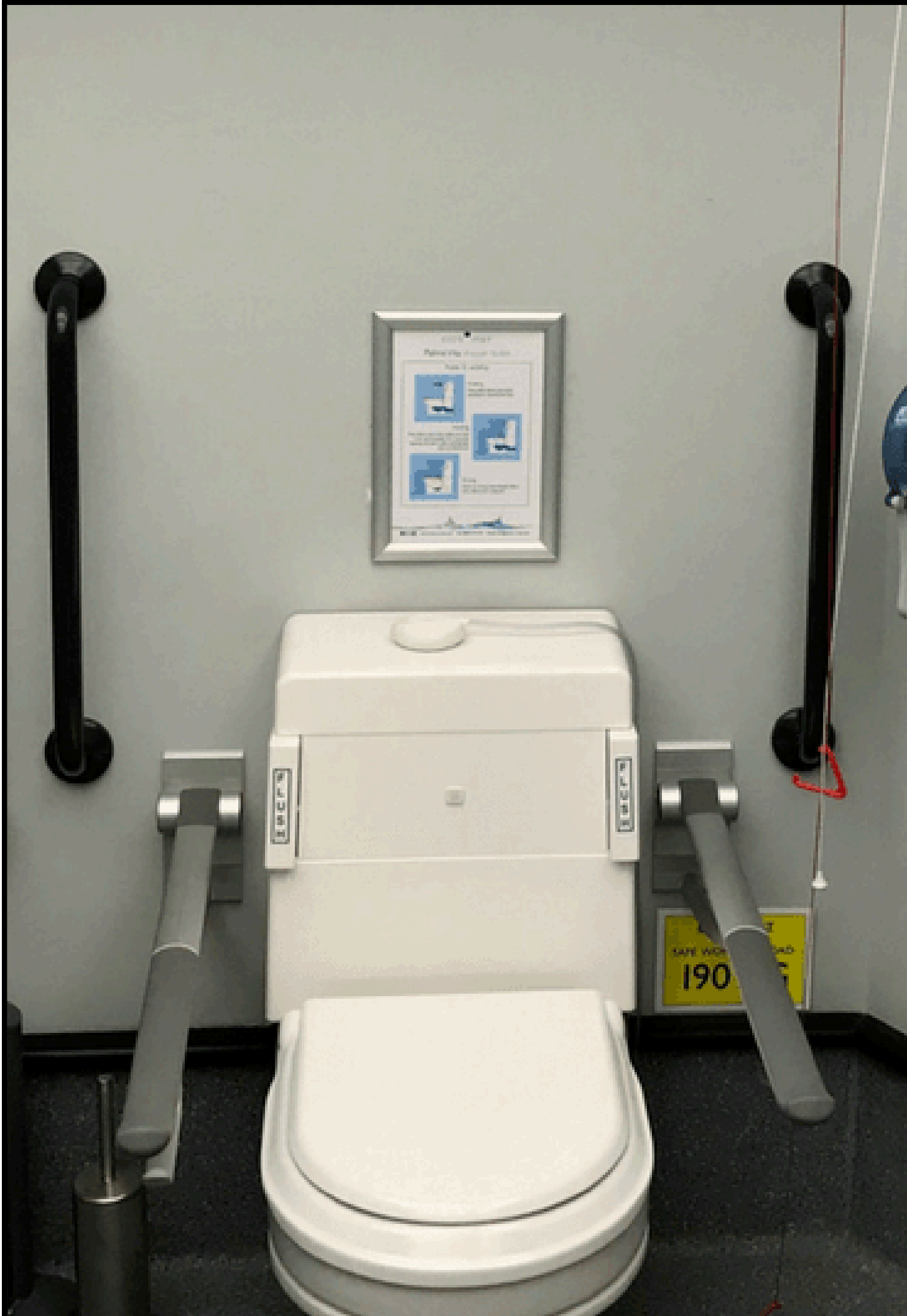
Figure 29 - Arts Building Changing Places toilet providing accessible facilities and space to support users with complex needs.
