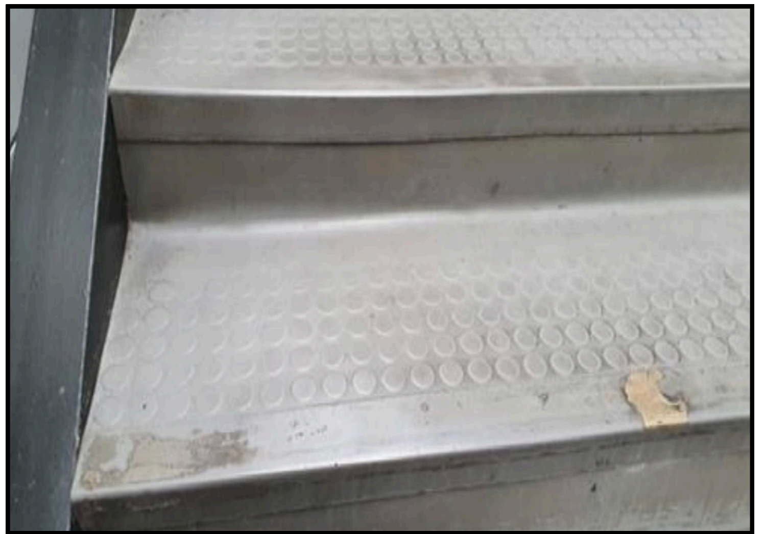
Figure 34 - Close-up of Main Atrium staircase with worn tactile strips and low contrast edges. Main atrium staircase has worn tactile strips and lack clear colour contrast at the top and bottom of steps, reducing accessibility for visually impaired users (Figure 34).
