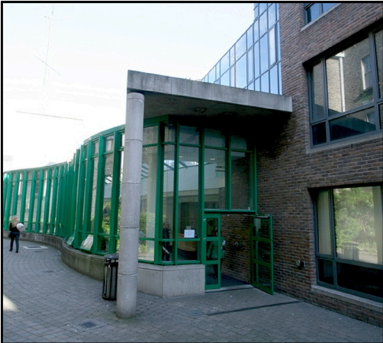
Figure 8 - Step-free entrance to Áras an Phiarsaigh with a clear, accessible route and automated door entry supporting independent access.
