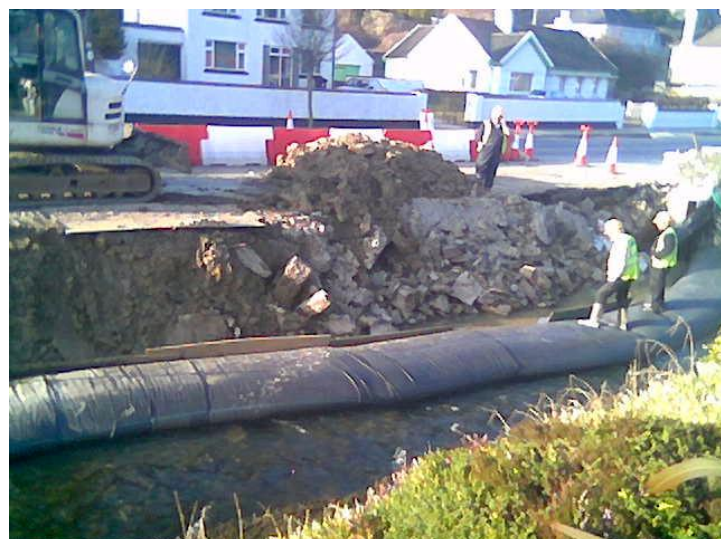
Plate 5: Aquadam in place for road reconstruction works (Photograph: Lisa M. J. Dolan courtesy of Atkins).
