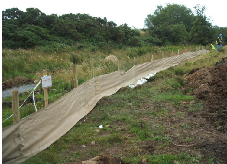
Plate 7: Silt fence under construction parallel to a 1 st Order River Nore tributary (Photograph: Lisa M. J. Dolan courtesy of Atkins).
