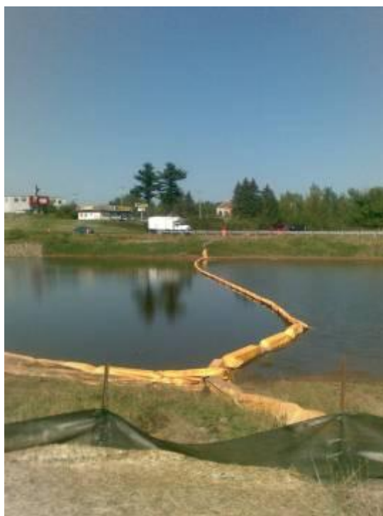
Plate 6: Pollution containment and silt fence within an attenuation pond in Minnesota state (Photograph: Lisa M. J. Dolan).
