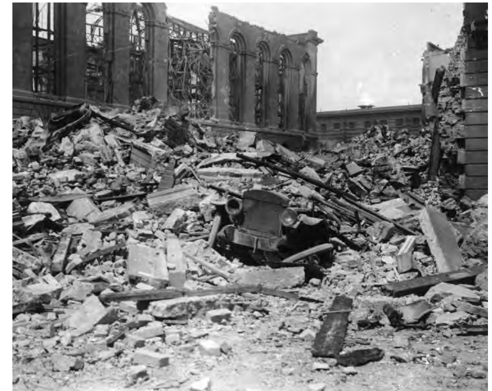
The remains of the Irish Public Record Office following the 1922 fire. (C/o of the Beyond2022 project)
