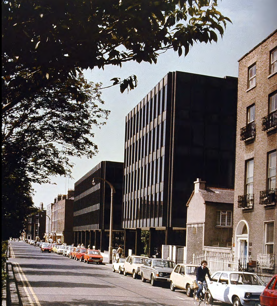
Scott Tallon Walker Bank Of Ireland Headquarters Baggot St Dublin 1968-72, 1973-75 Exterior
