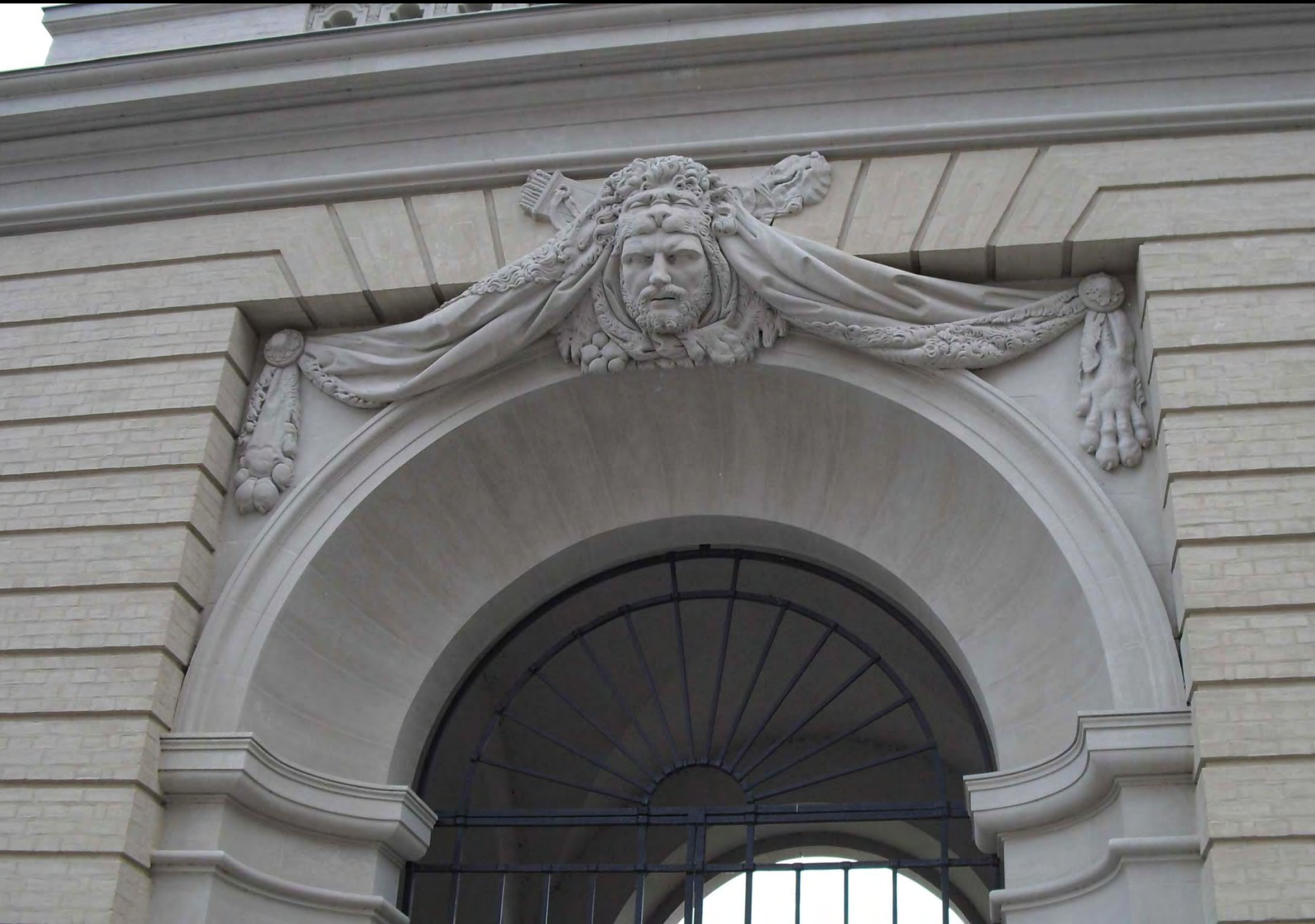
Palace Gate, Potsdam, Prussia c.1700
